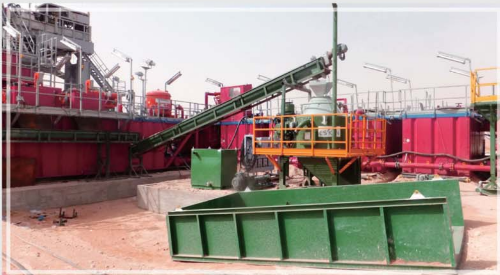
KOSUN VC-1000 Operating on drilling site
